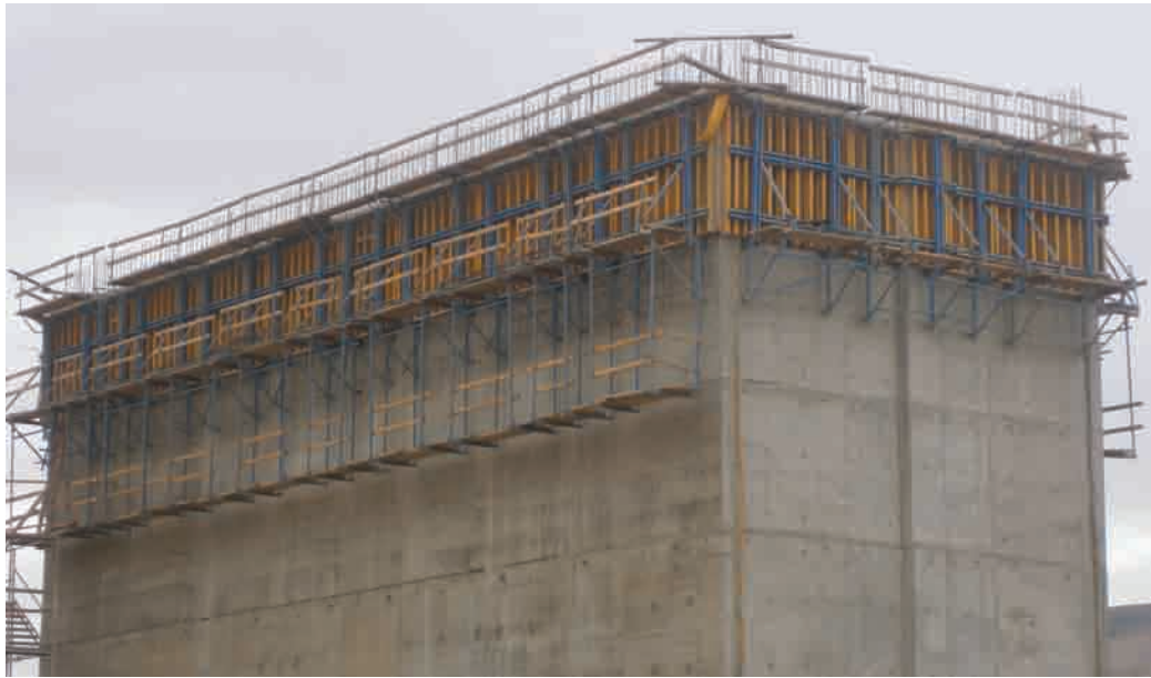
Concrete weight blocks for anchoring the push-pull props.
