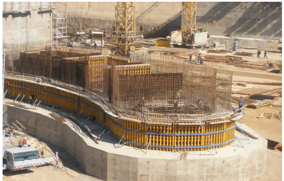
Slight curvatures with SIMPEX at Cheliff Dam
