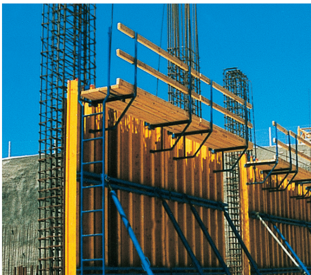
Access ladders and working platforms with SIMPEX.
