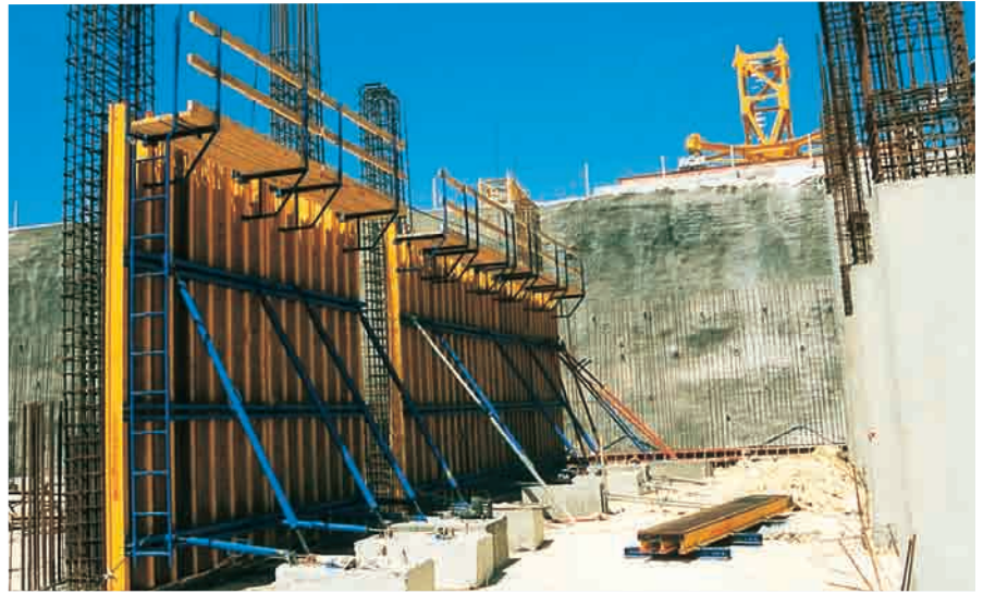
Concrete weight blocks for anchoring the push-pull props.
