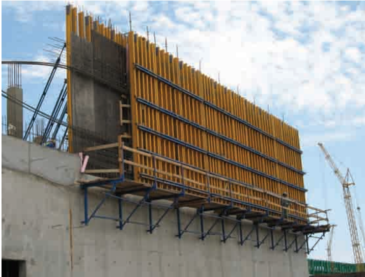
SIMPEX Formwork at an industrial job-site in KAZAKHSTAN.
