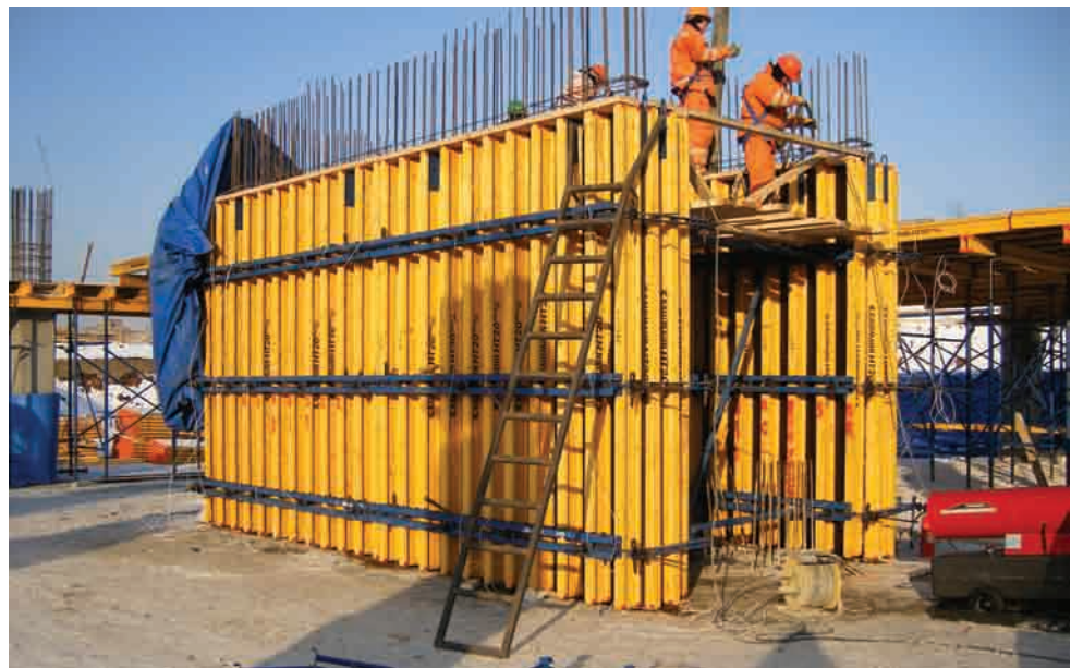
SIMPEX Formwork at an industrial job-site in KAZAKHSTAN.
