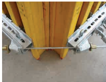
Corner-shoe detail for angular corner tensioning
